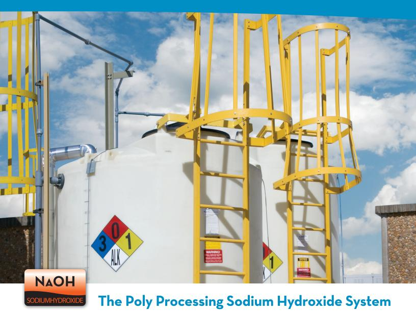
The key to storing sodium hydroxide properly is strong, safe containment. Since the chemical is so corrosive, secondary containment is an absolute.
